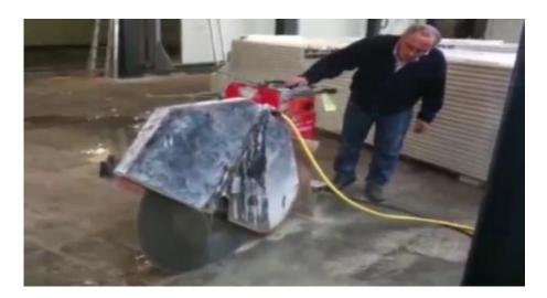
Here is the tool which is used today to pierce a squared hole in a concrete slab, 20cm deep. You can see how difficult it is! Another tool can also be used which is much less bulky.
